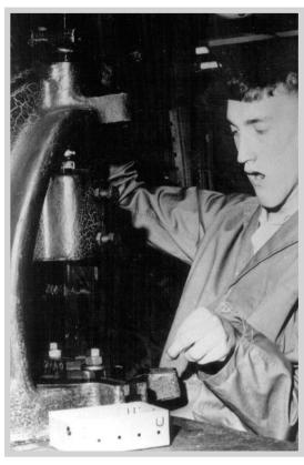
Adrian Lynch operates a large handpress which involves control finger movement to place a component in the die.
